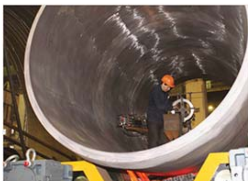
Overlaying welding of the inside surface of a shell
